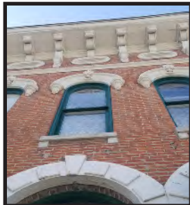
2.a.iv. Roof features and detailing are key characteristics of the Downtown District.
